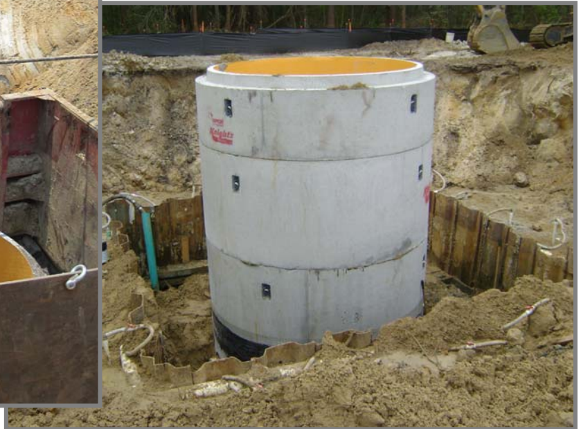
Pipe for ISM Group 2 gravity sewer and construction of PI 08 wet well.
