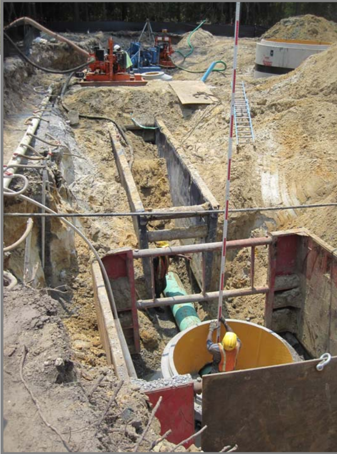
Pipe for ISM Group 2 gravity sewer and construction of PI 08 wet well.
